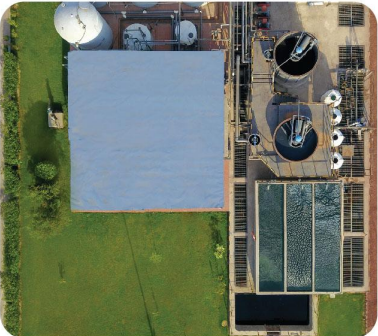
ETP (60m 3 /hr) & recycling (60% efficiency)
