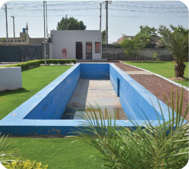
Rainwater harvesting (12000 gallons)
